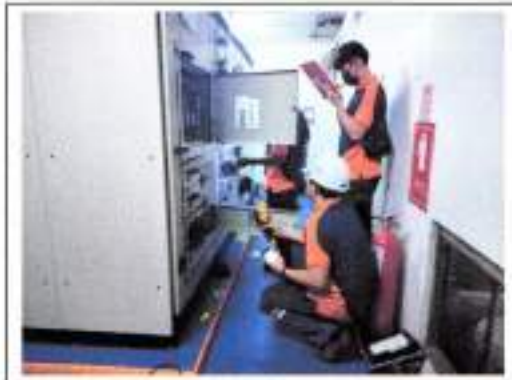
Picture 4: Main distribution board and preventive maintenance.
