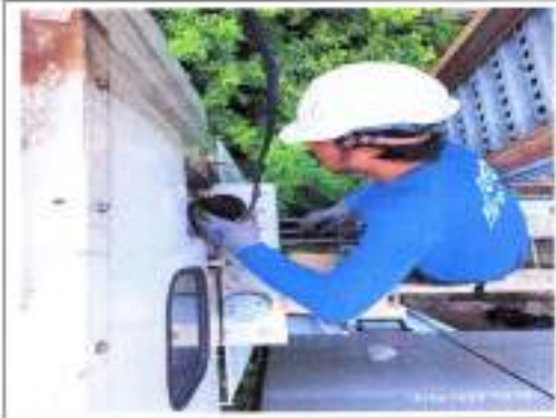
Picture 2: Electrical part replacement. (Thermometer transformer)
