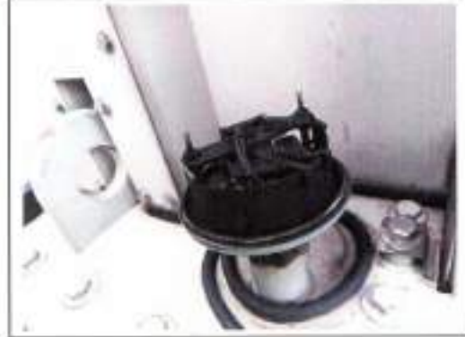
Picture 2: Electrical part replacement. (Thermometer transformer)
