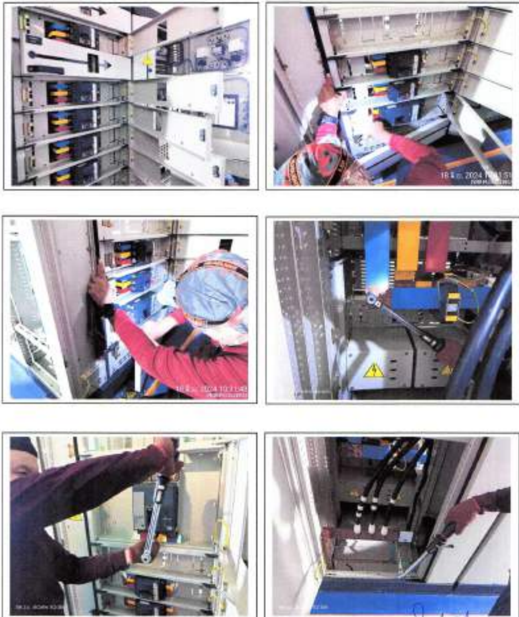
Picture 3: Main distribution board and preventive maintenance.
