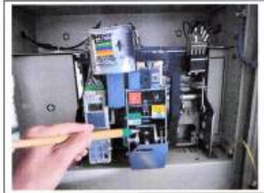
Picture 5: Air circuit Breakers and preventive maintenance.
