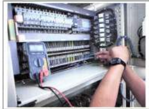
Picture 4: Main distribution board and preventive maintenance.
