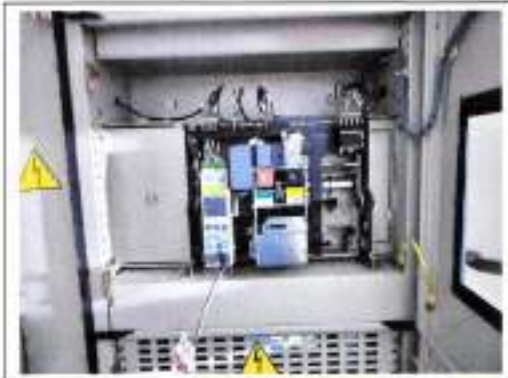
Picture 5: Air circuit Breakers and preventive maintenance.
